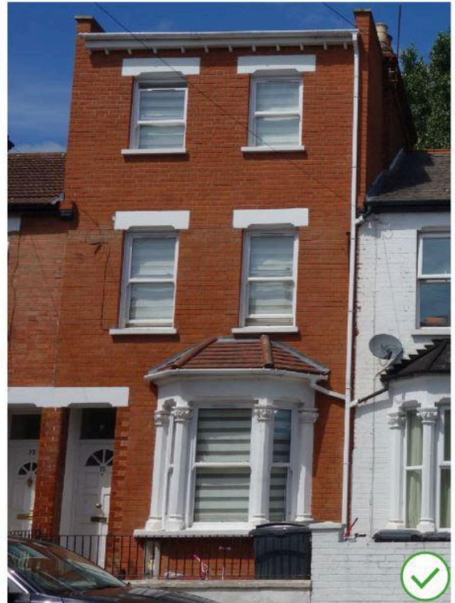
Fig.25: The external design of the new top storey extension matches the design of the existing house with aligned matching windows, flush facade and matching brick detailing that continues seamlessly
