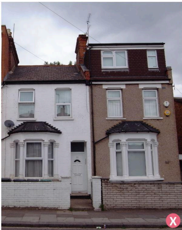
Fig.21: Dormer windows not set back from the roof eave and not set in from the party wall, windows misaligned from the existing windows below
