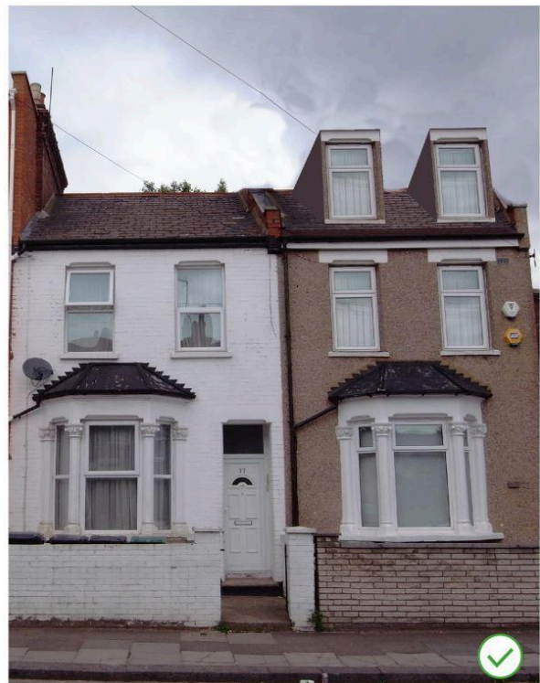
Fig.22: Dormer windows set back from the roof eave, set in from the party walls and aligned with the existing windows below
